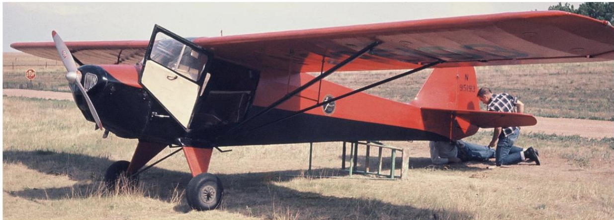
Taylorcraft BC-12D (95193) circa Sep/Oct 1963 at Fountain Airport. Nick Lacey and unknown person are repairing the tailwheel. Note the sophisticated jack-stand. (Photo by Gary Dickinson '64)
